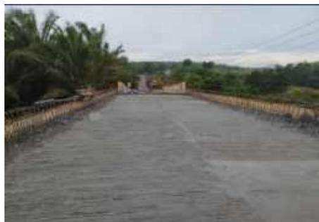
Gambar 4 Perkerasan Beton Semen
