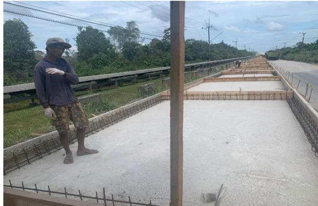
Gambar 6. Pemasangan bekisting beton mutu Fc 30 Mpa
