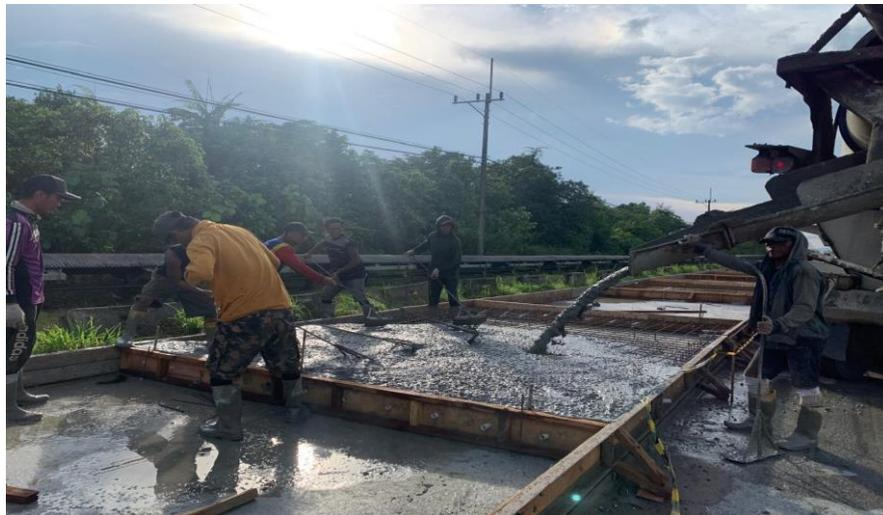
Gambar 8. Proses pengecoran beton mutu Fc 30 Mpa
